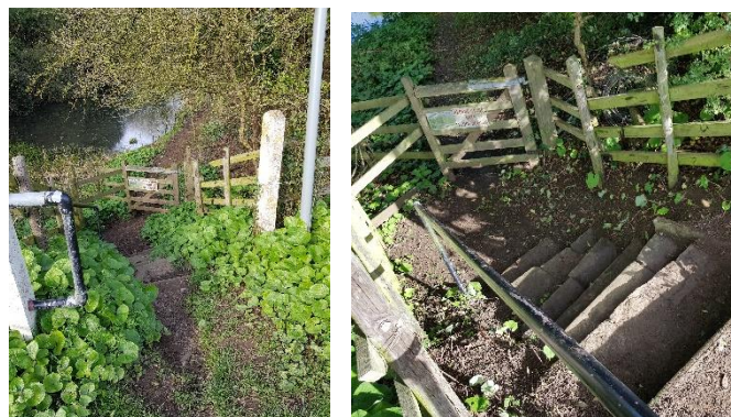
Vegetation removed from the northern section steps
